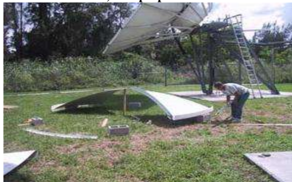
Professional installer begins assembly of an Andrew 4.5m
