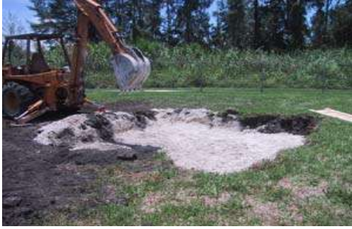
Excavating the whole for the antenna
