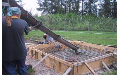
Building the concrete pad
