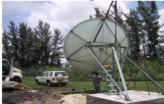
Installing the antenna on the support frame
