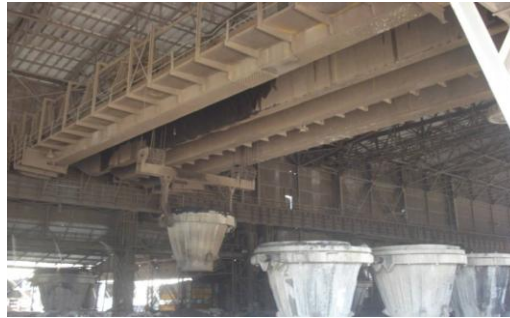
Fig.7 Crane dumping of slag pot
