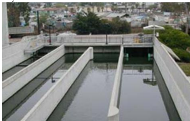
Figure 1: settling tank in Effluent Treatment Plant
