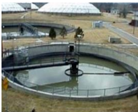
Figure 4: aeration tank in a Effluent Treatment Plant
