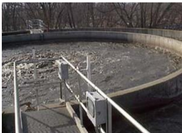
Figure 2: equalization tank in Effluent Treatment Plant
