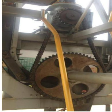
Figure 3: Actual chain system at the garage
