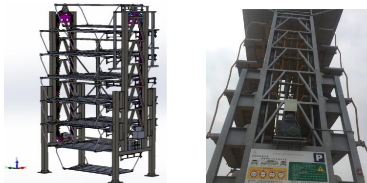
Figure 1: 3D Structure of the vertical stereo circulation garage.
