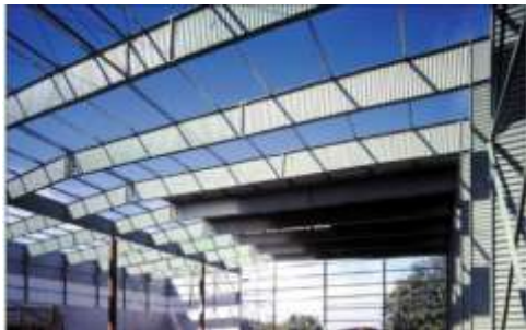
Figure 4. Corrugated web girder in industrial buildings
