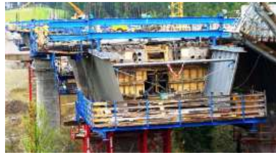
Figure 5. Corrugated web girder in Bridge construction
