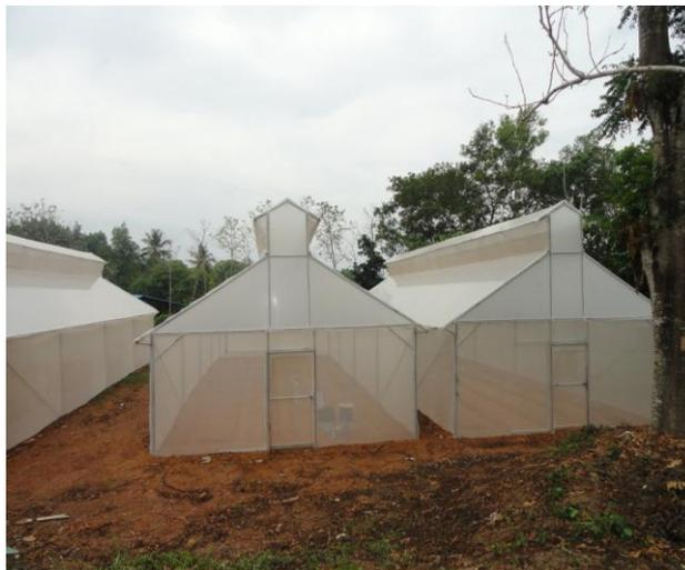
**Fig.1: Naturally ventilated Gable type poly house structures**
