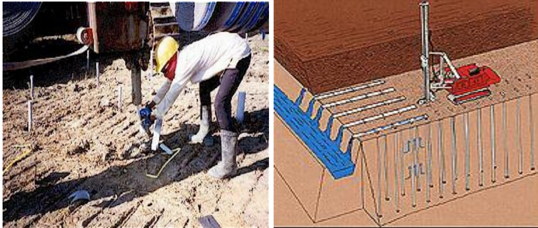
Fig. 2 Installation of drain.
