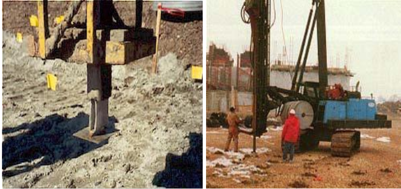
Fig. 1 Installation equipment for wick drains.
