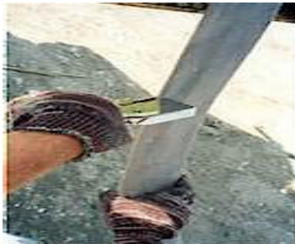
Fig. 3 Splicing of wick drains
